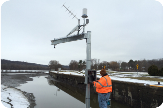
Xylem representative installing a HydroMet monitoring solution
