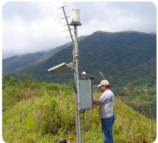
Turn-key monitoring station containing a YSI Rain Gauge, Storm 3 Data Logger, GOES telemetry, and meteorological sensors.
